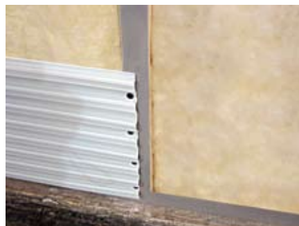
2 #1033 - Primary Insulator, fastened horizontally to the studs
